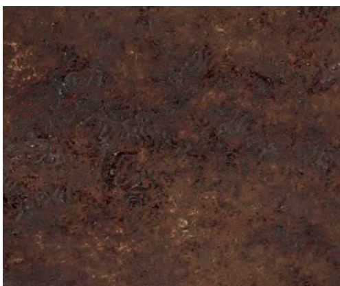
Metal rust - Red
